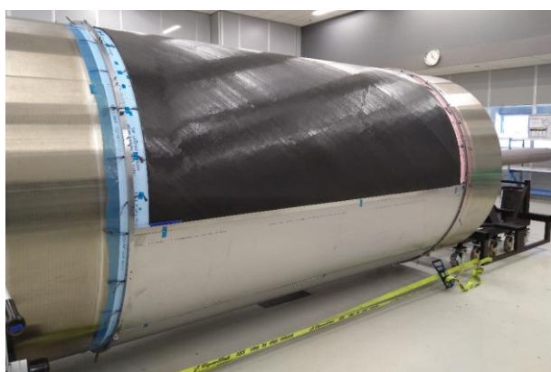
Figure 8: Caul plate installation after skin layup.
